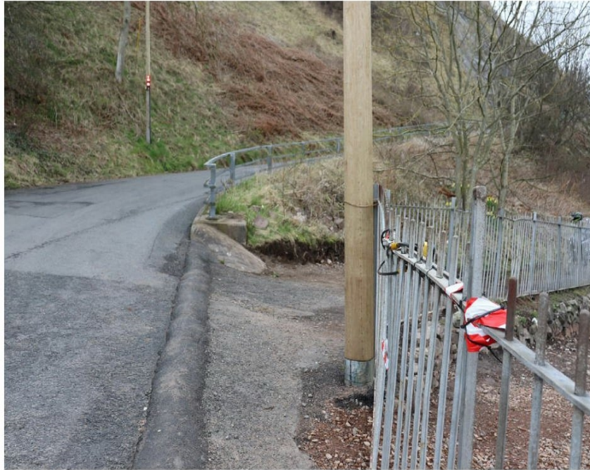
Figure 9.0 – Raised Road Surface.
